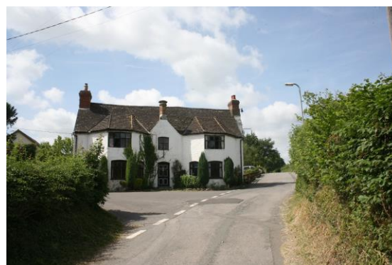
Fig.38 Hostry House terminates views from the White Castle brook
