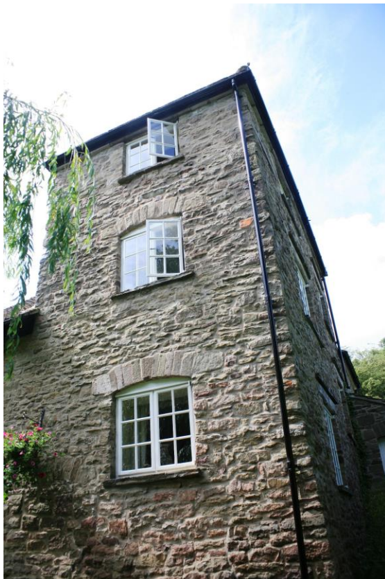
Fig.41 Characteristic rubblestone walls at Llantilio Mill
