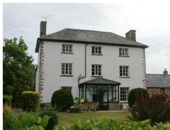
Fig.50 White House Farmhouse. A strictly symmetrical early -18 th century farmhouse, with sash windows on the ground floor and casements above. The central porch is modern
