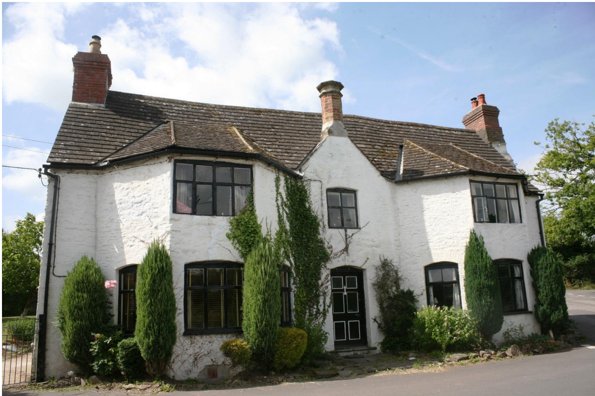
Fig.48 Hostry House. A wide fronted house, much altered but with 16 th century origins, located in the centre of the village. The central gable chimney and shallow canted bay windows are unusual features
