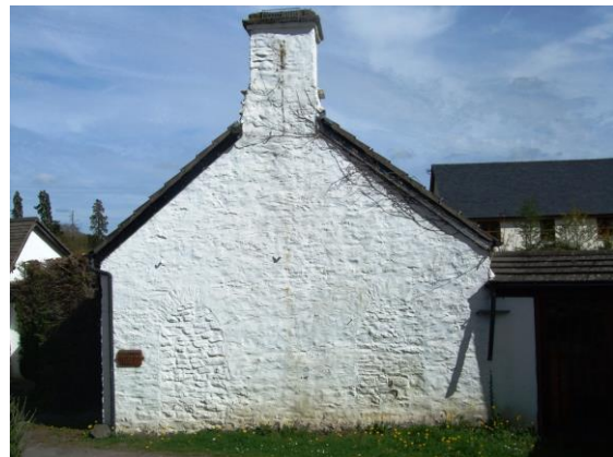
Fig.34 Paired blocked archways in the gable of Hostry Hall
