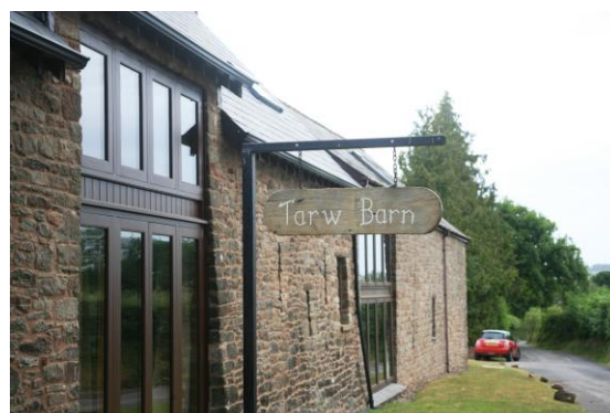
Fig.45 The Barns at White House Farm are attractive, converted traditional farm buildings but retaining many of their external characteristic features
