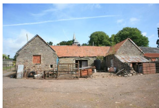
Fig.52 Court Farm. A fine U-plan stable range with an unusual canted drip mould lintel. The pantiled roof is a colourful contrast to the natural slates on almost all the buildings in the village
