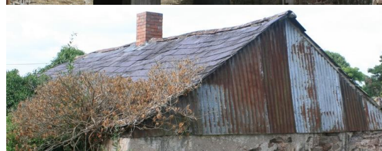
Fig.58 Examples of roof materials used in the Conservation Area
