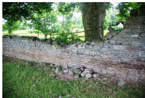
Fig.15 Coursed sandstone rubble walls are a feature of the former Court grounds
