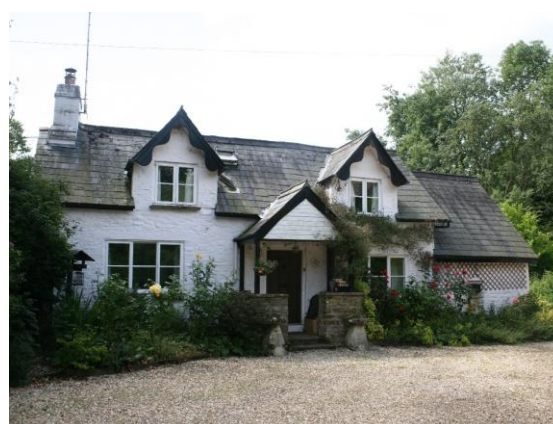
Fig.46 Cottage near the former Water Mill. Its basic form is that of a vernacular dwelling although it appears to have been adorned with later Victorian additions including the decorative bargeboards
