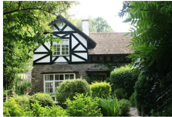
Fig.55 Raglan Lodge. A late 19 th century estate cottage. A decorative half-timbered first floor and projecting bay windows feature in this deliberately picturesque composition
