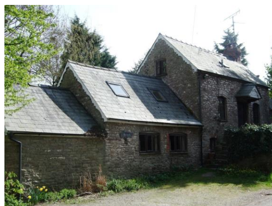
Fig.44 Former Blacksmiths. A typical vernacular composition of main building and secondary wings set out in linear fashion and of diminishing heights.
