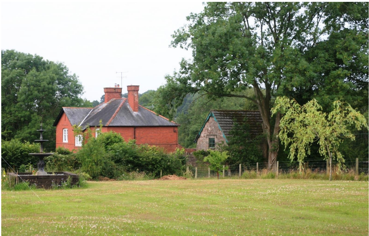
Fig.35 The red brick vicarage and stone outbuilding survive and form a significant group
