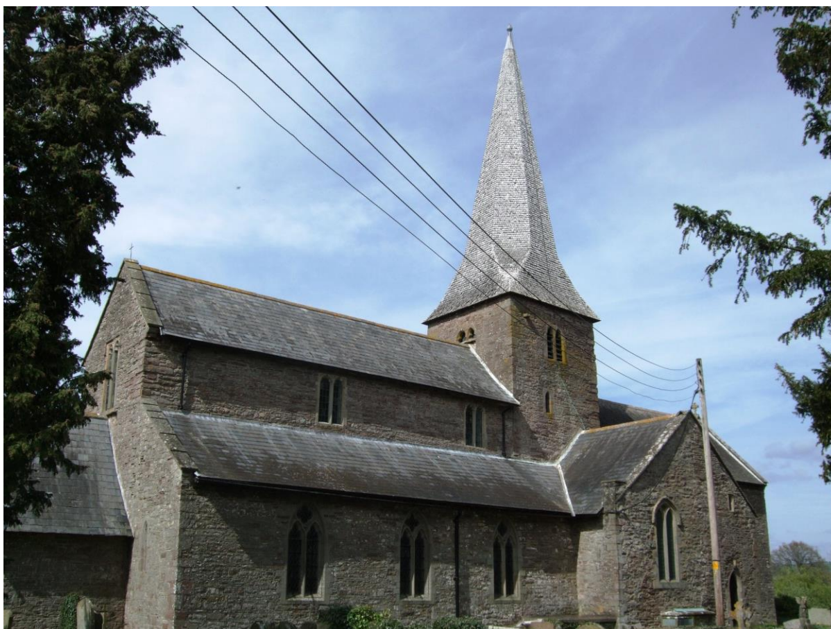
Fig.47 St Teilo's Church, a magnificent mainly 12 th century cruciform church with an 18 th century shingle-clad spire, is located in a commanding position in the village. The 15 th century raised clerestory and west window contribute to its striking profile
