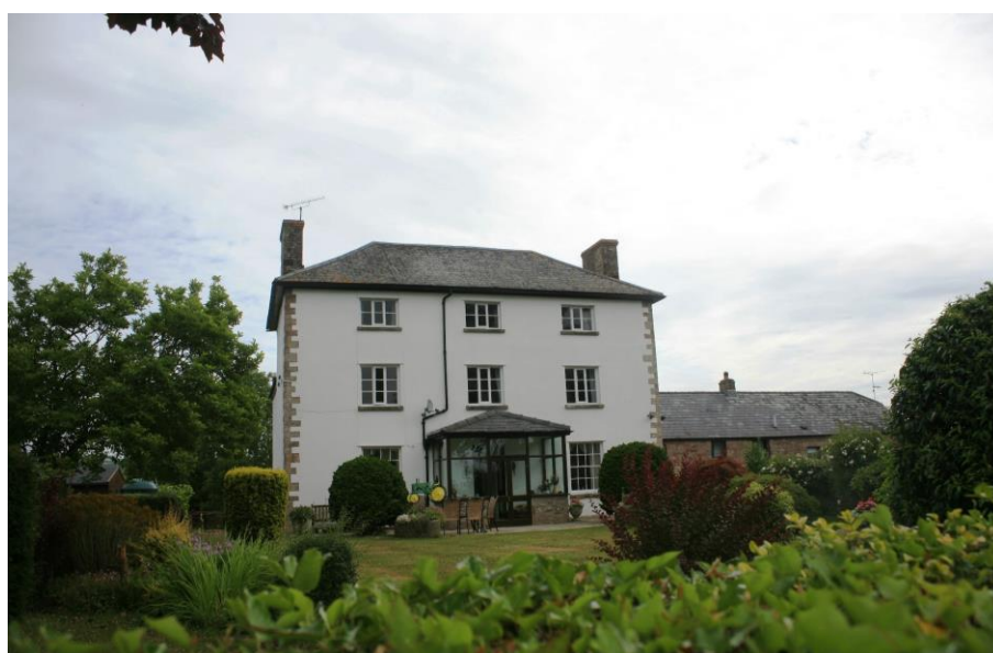
Fig.27 The formal symmetrical façade of White House farmhouse
