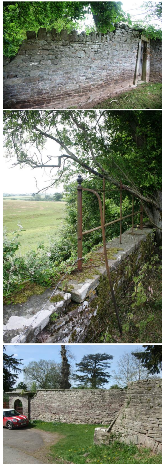
Fig.59 Examples of boundary walls and retaining walls within the Conservation Area
