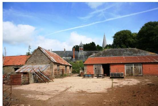
Fig.17 Agricultural buildings at Court Farm display a wide variety of materials including rubblestone, brick, clay tile, slate and corrugated iron
